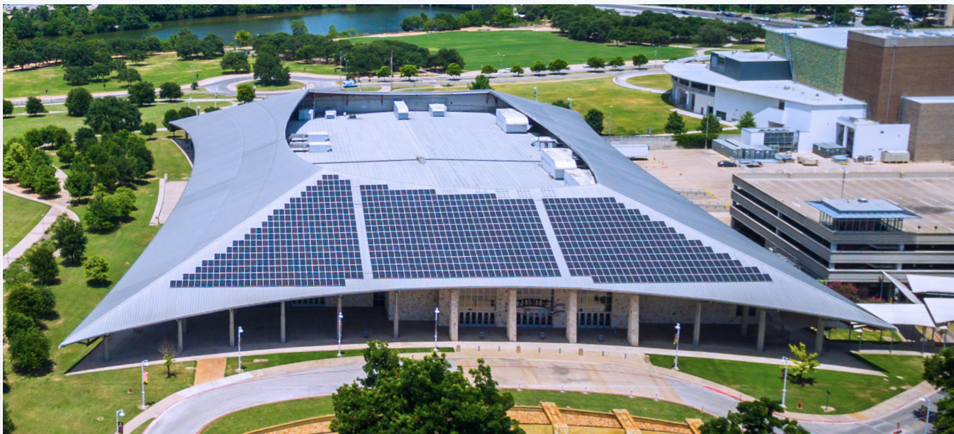
Local solar on the Palmer Events Center.
